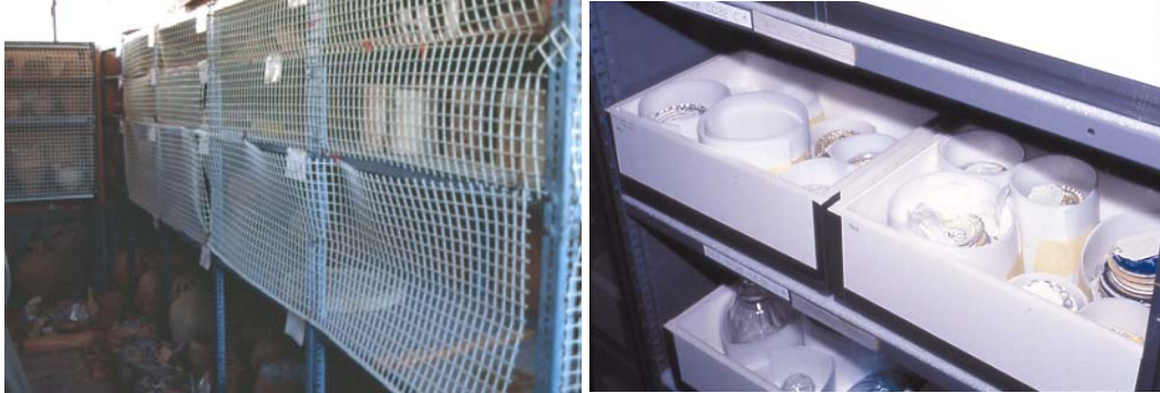
Sungay Fig. 1: On the left, inexpensive netting is secured across the front of these open-faced shelving units. The netting prevents vases on the shelves from falling to the floor during an earthquake. On the right, the use of thin ethafoam sheets to surround individual objects on shelves. The ethafoam prevents the objects from colliding into each other or rubbing against each other during an earthquake. The shelving units have also been secured to the wall and floor. (photos J. Podany)
