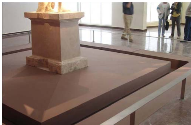
Koumouisis Fig. 3: The monumental marble statue of Hermes installed at the new Archaeological Museum in Olympia. The statue is isolated by a base isolation mechanism installed in a cavity built into the floor. On the right the supporting platform, on which the statue and its pedestal rest, is shown. Note the sufficient space between the edges of the platform and the protective rail that surrounds the exhibition assembly to accommodate the lateral displacement of the base isolation unit (and sculpture).
