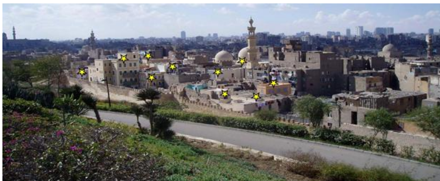
The cumulative results of an integrated program of urban rehabilitation Darb al-Ahmar, Cairo (2000-2009). Photo: Francesco Siravo
