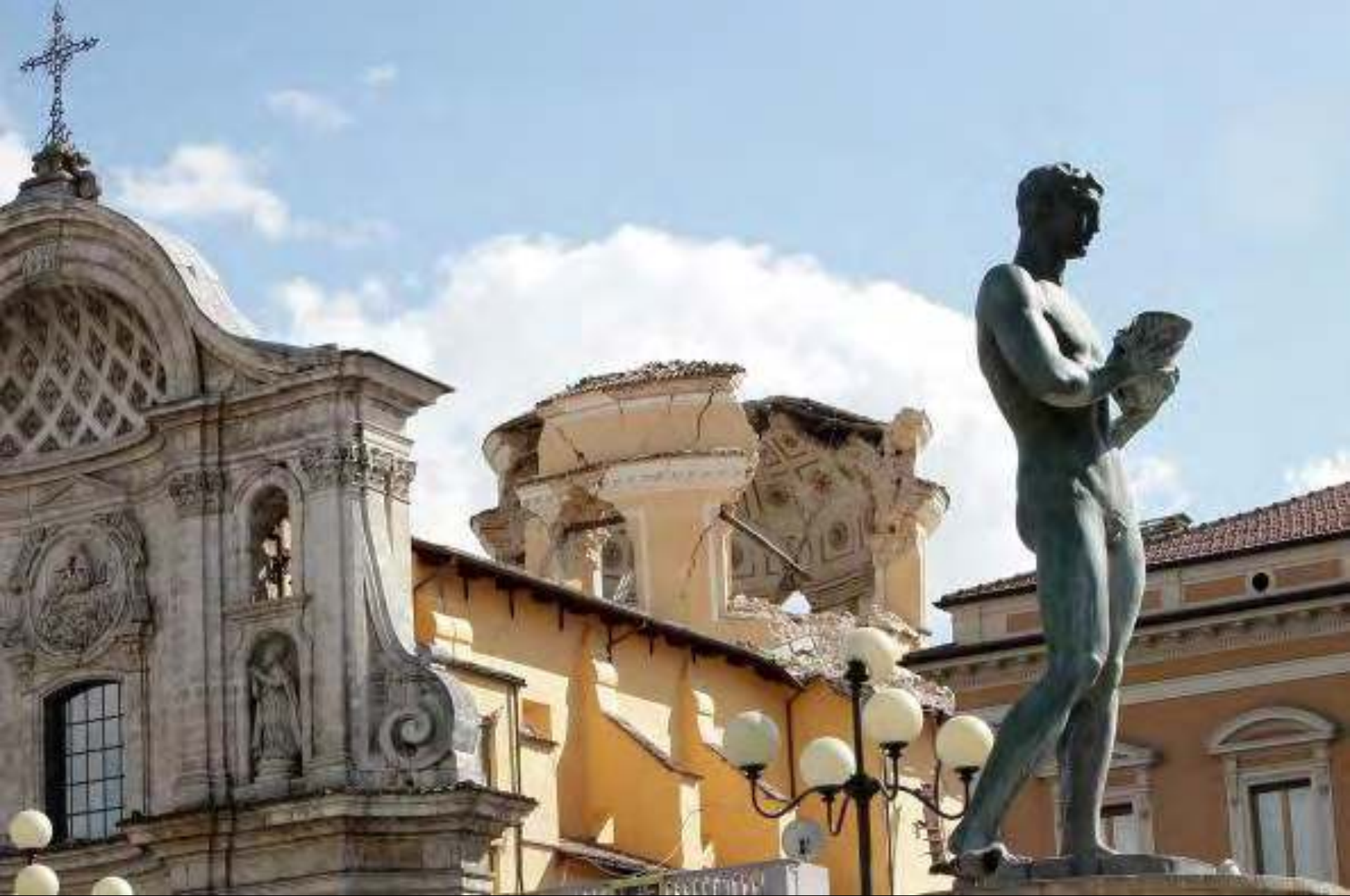
L'Aquila earthquake : 6 April 2009
