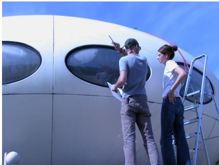
Futuro house, Matti Suuroonen, 1968, Investigation of glass-fibre reinforced polyester surface, photo: Tim Bechthold, copyright: Die Neue Sammlung. The International Design Museum Munich.
