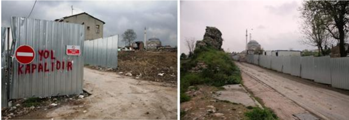
Sulukule today, as a construction site. Photo: Najila Osseiran
