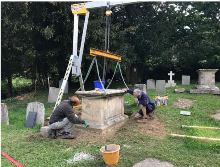
FIGURE 1. Churchyard of St Cyr, Stinchcombe. Graham O'Hare (right) with a member of his team, reinstating the lid of the table tomb of Mary Manning. Image: Adam Klups
