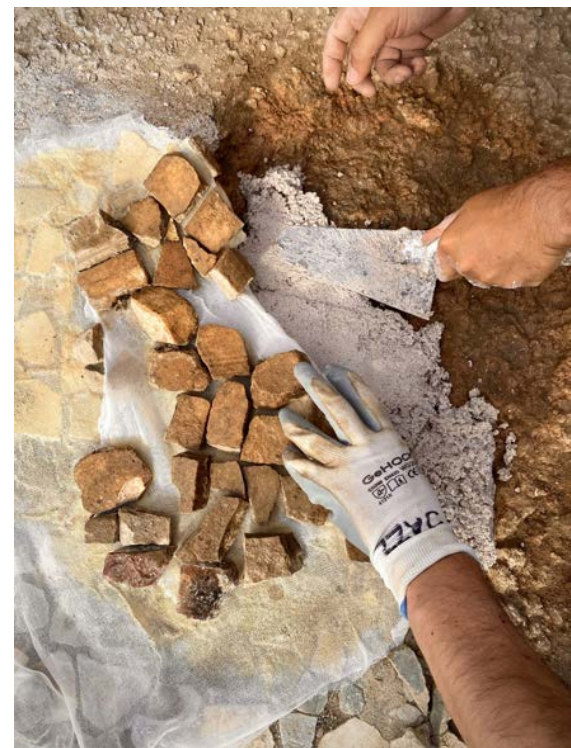
New mortar being laid under a section of mosaic that has been supported and lifted using a gauze facing and adhesive facing. Photo @ Shoun Obana
