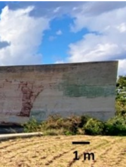
The concave, north-facing side of Il-Widna shows the five coloured camouflage paints: green, red, yellow, light brown, and dark brown. This photograph was taken with a wide-angle lens, so the scale is slightly skewed. © Ruiz 2021
