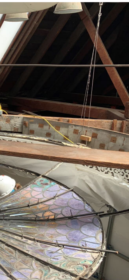
Above: On site shot of the Nzilani team removing an inverted stained glass dome. Makau in green hard hat. Photographer: Nzilani.
