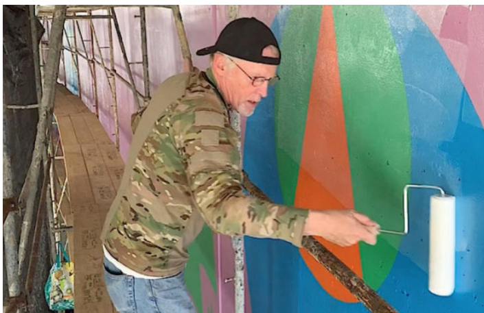
Scott Haskins applying the final varnish anti-graffiti protection layer. © FineArtConservationLab.com
