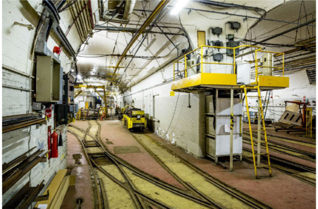
Exhibition Space and Controller's Platform from Entrance to Orientation and Events Space.jpg Miles Willis Photography © The Postal Museum (2018)
