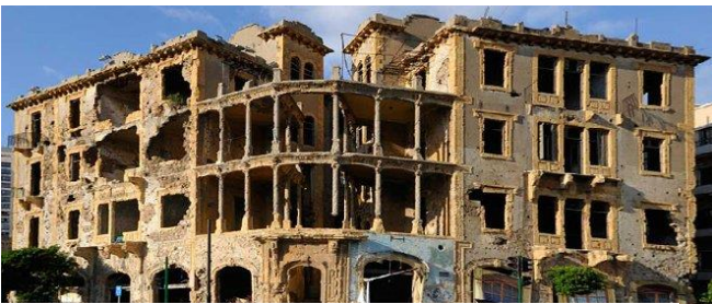
Barakat House, Beirut, before restoration
