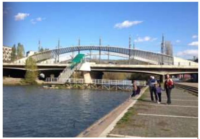
The bridge is barricaded by rubble on the north side
