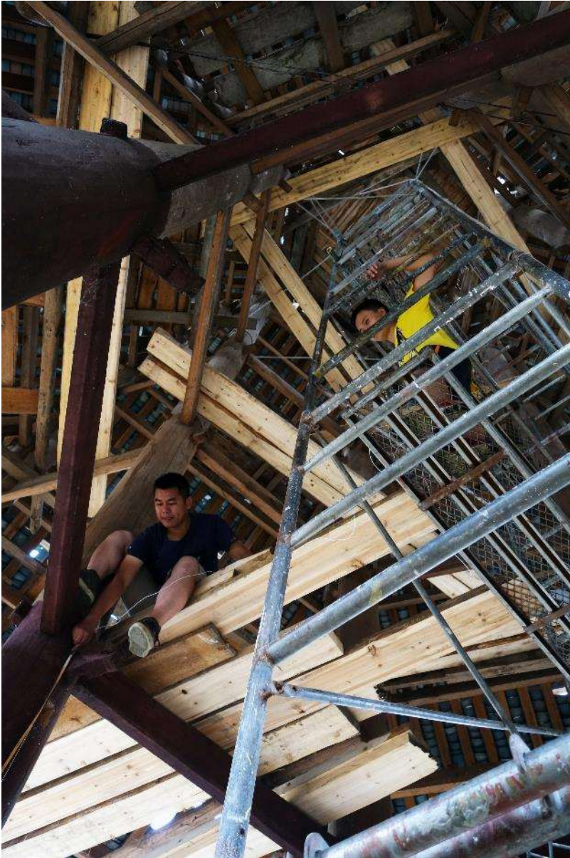
Assessment of the drum tower structure
