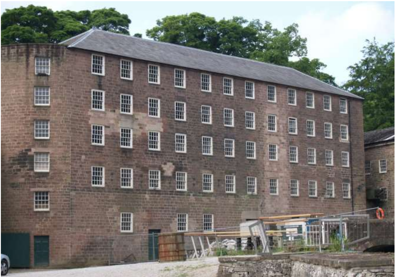
Exterior view of Building 17
