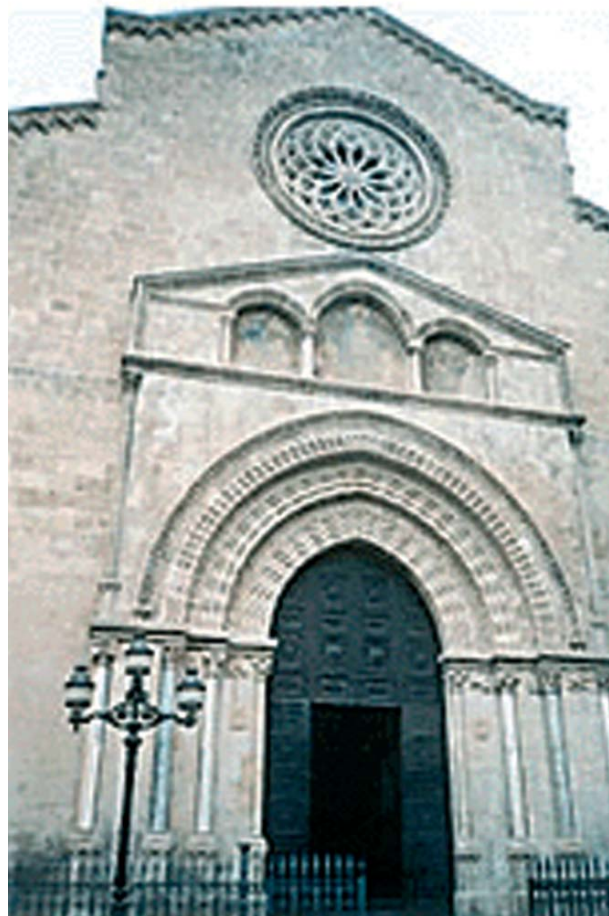
The façade of the Church
