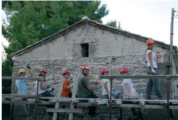
Removing the cement joints
