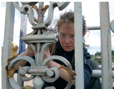
Jo Adkins removing paint to expose hidden corrosion
