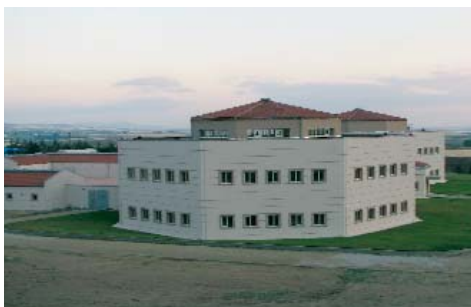
Octagonal building in foreground housing the conservation laboratory
