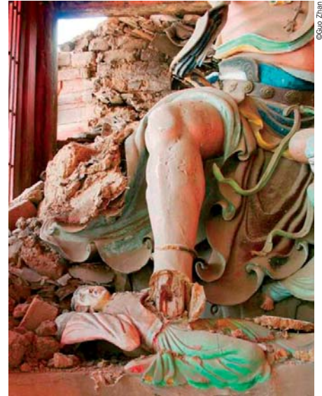
Baoren Temple in Pingwu county, Sichuan province after the earthquake.
