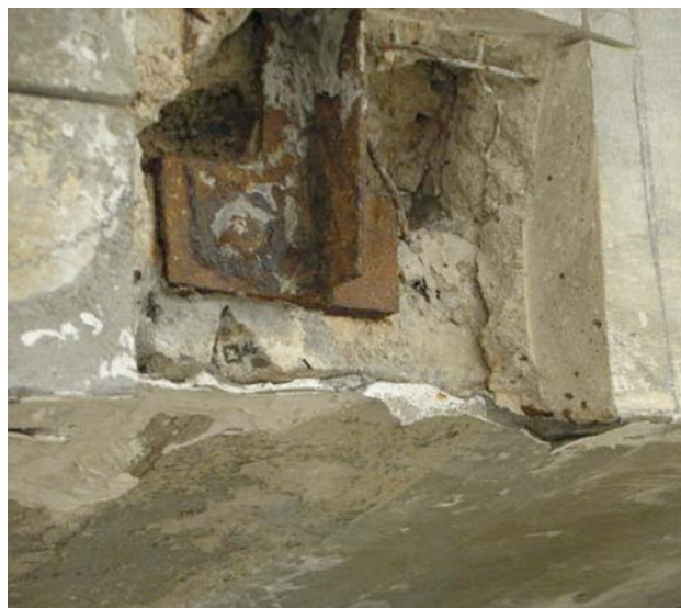
Probes revealed corrosion of the embedded steel T-shaped beams
