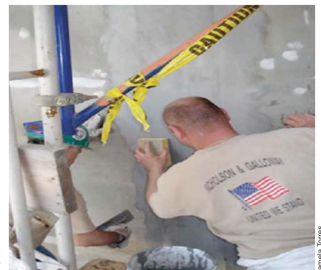
Mock-up of treatment of severe cracking on 6th ramp
